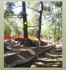
Log walls (above) were backfilled in lifts with selected soil material placed carefully around roots. A new slope was created providing space for healthy root systems to reestablish.
