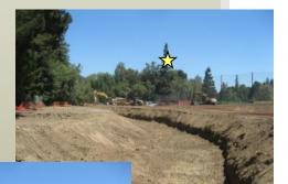
During construction, the new channel was excavated. Cobbles and gravels were used to create the new creek bed.
