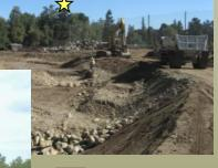
The brand new creek, shown photo left Dec. 2008, was created where parking had existed. The new channel allows for desirable in-stream floodplain "benches" and supports greater habitat complexity. The channel slope is gradual and there are no longer barriers to fish migration.
