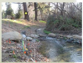
A new pool was created below the boulder cross vane. The cross vane will stabilize the channel bed at the proper elevation and maintain the improved fish passage conditions.
