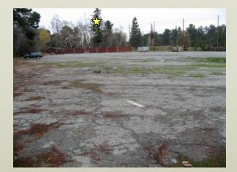
The lower portion of the former parking lot shown in photo left was removed. It became part of the new creek channel, allowing creation of a wider, stable and healthy channel configuration.
