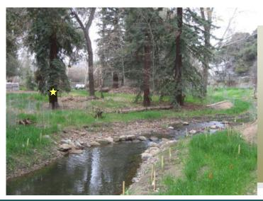
The creek restoration removed the low flow structure and riprap. The redwood tree marked with a star in the upper photos is the same tree marked in this postconstruction photo left. A boulder cross vane helps stabilize the channel bed and create a pool-glideriffle sequence.
