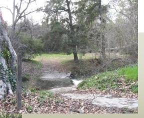
The first low-flow crossing was a driveway through the creek to Fallen Oak picnic area. Its presence created a vertical drop, causing problems for
